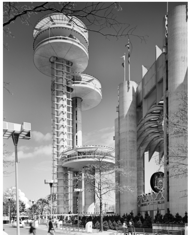
Figure 15 Philip Johnson, Skystreak elevators, New York State Pavilion, New York World's Fair, Queens, 1964 (© Ezra Stoller/Etso).
